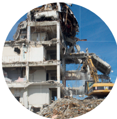
Construction & Demolition Waste
